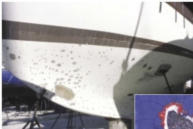
Spot-repairing blister domes by grinding and filling with epoxy or resin is strictly a cosmetic approach. The problem remains, and new blisters will continue to form.
