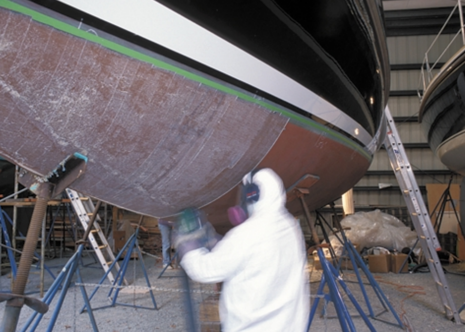
A fiberglass peeler at work. Sometimes the only solution to blisters is removal of several layers of fiberglass from a hull.
